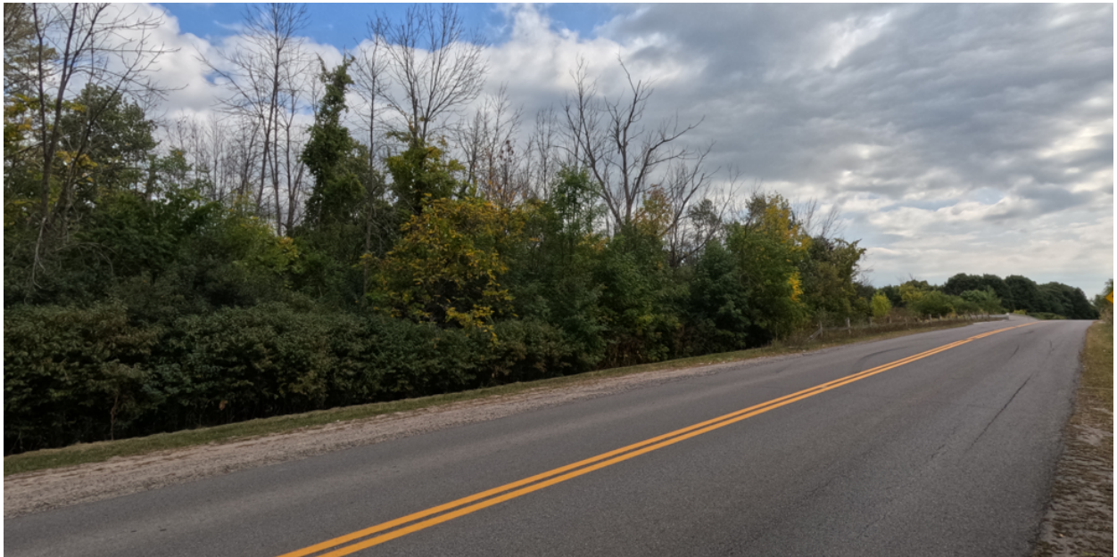
Figure 5: Forest Buffer Between Concession Road 2 and Highway 401
